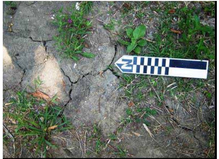
Figure 1: Typical view of levee clay shrinking as it loses moisture (and cracking as it loses volume). This photo was taken May 23, 2011, on West Bank MRL, downstream of Algiers Point (Maritime Navigation) Light.
