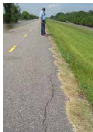
Figure 7: Inferred tension crack in levee crown above Drifting Post #6 and new cracks. Flood Authority Superintendent Mr. Chris Muscarello stands at the end of the inferred tension crack seen in the foreground.
