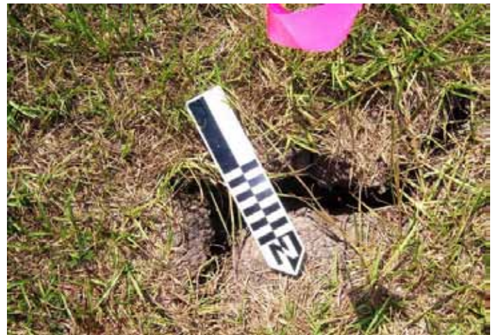
Figure 2: Excessive cracking downstream of HPL Bridge on West Bank MRL.
