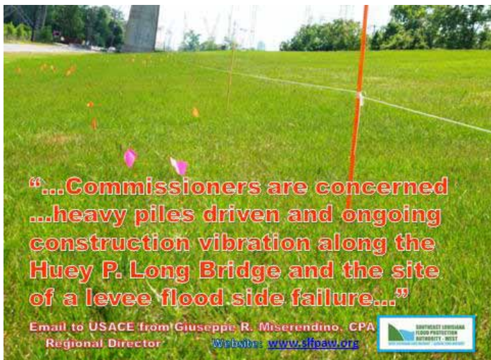
Figure 9: Cracks flagged by Southeast Louisiana Flood Protection Authority-West (SLFPA-W) inspectors. Note Huey P. Long Bridge pier in background is aligned with crack trend.
